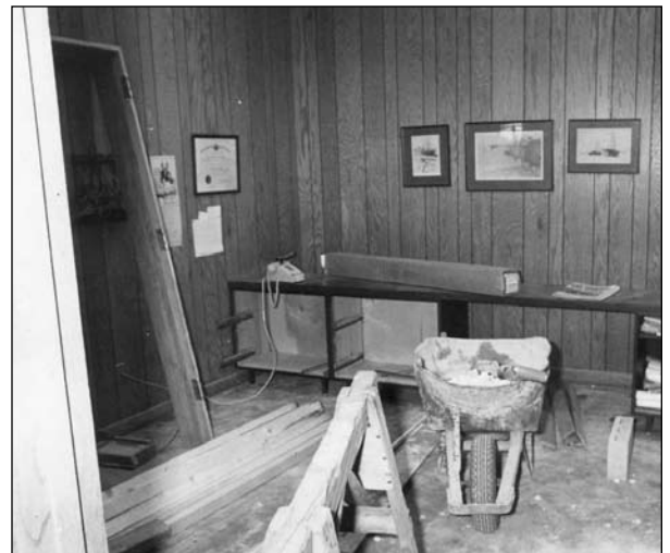
Alterations to the circulation desk and office area of the library were made in 1977.
